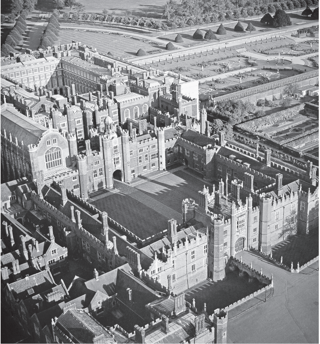
Hampton Court (zestiende eeuw). Uit: P. Henderson, The Tudor House and Garden: Architecture and Landscape in the Sixteenth and Early Seventeenth Centuries , New Haven (Conn), 2005, 41.
